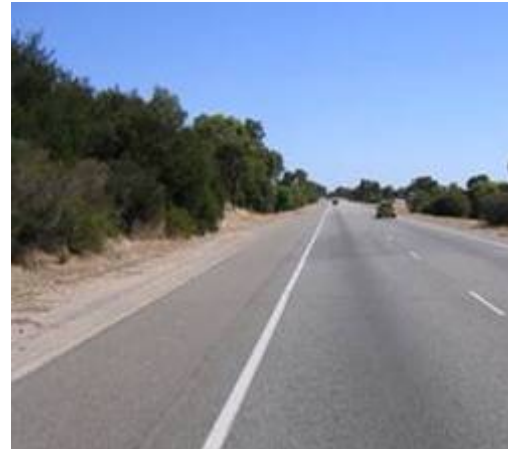
Shoulder sealing with edge lines
