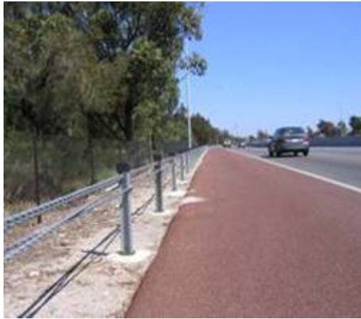
Wire rope barriers
